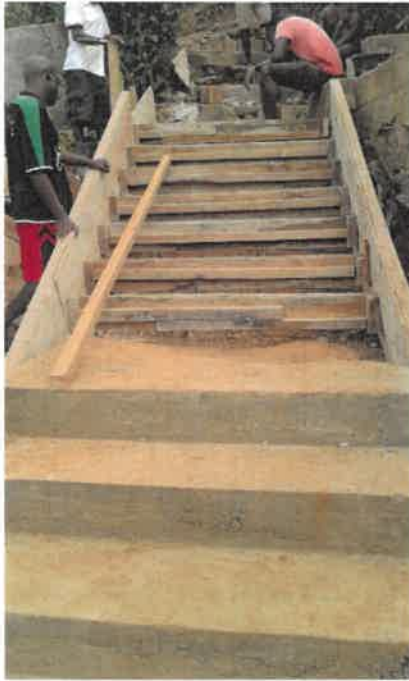
Figure 1: Construction of Stairs in Progress
