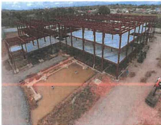
Decking Installation – South East View
