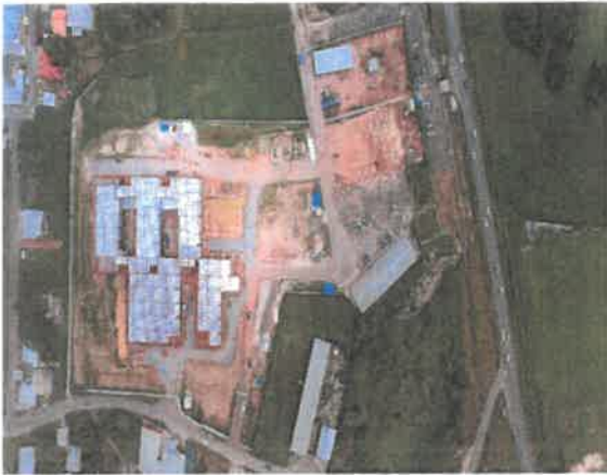
Overview of works onsite
