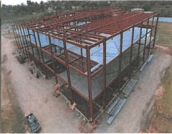
Decking Installation – North East View
