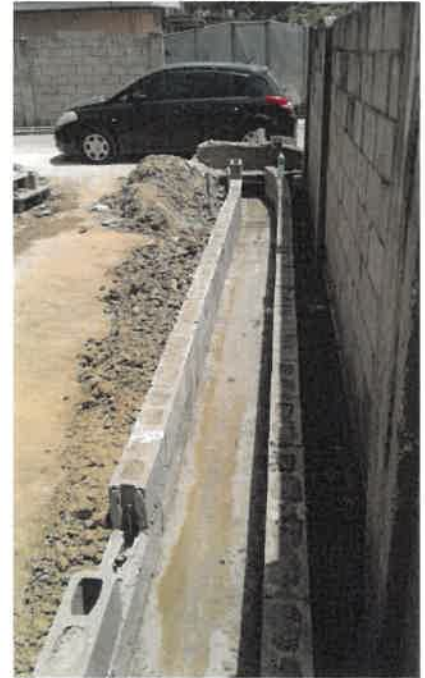
Figure 2: Construction of Box Drains
