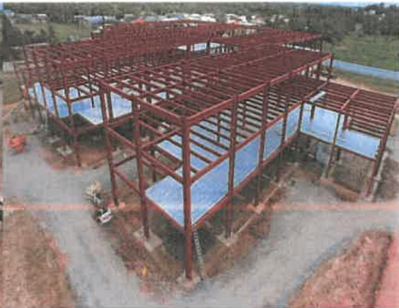
Decking Installation – South West View
